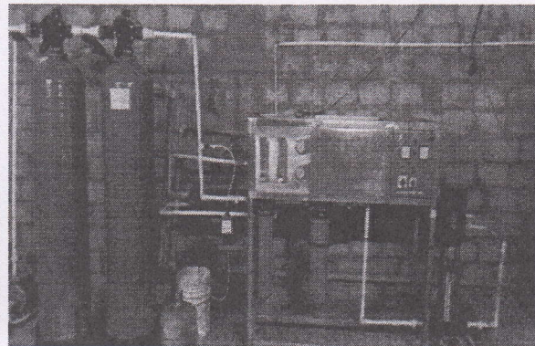
RO water plant arrangement in the campus
