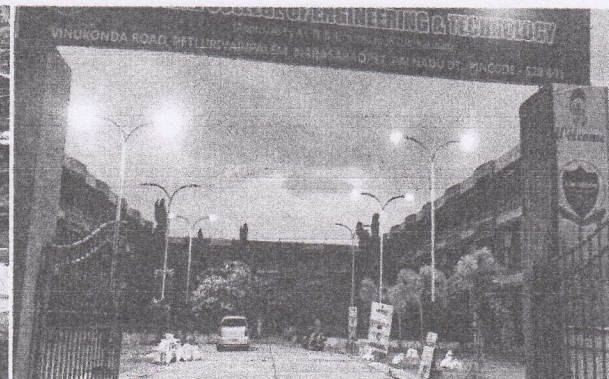
LED street lights at the entrance gate
